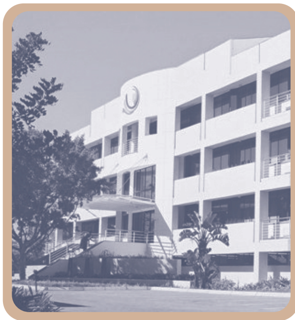
New Head Office Building, Erasmusrand
